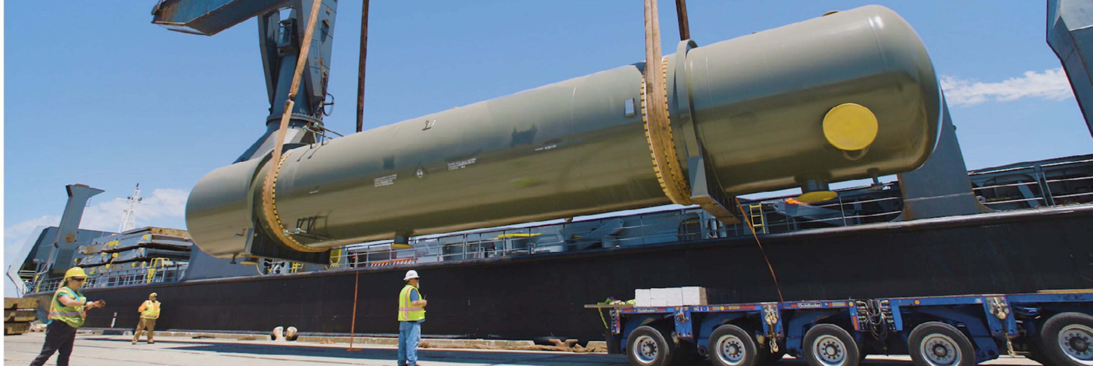
CD4 Power Plant constructions
