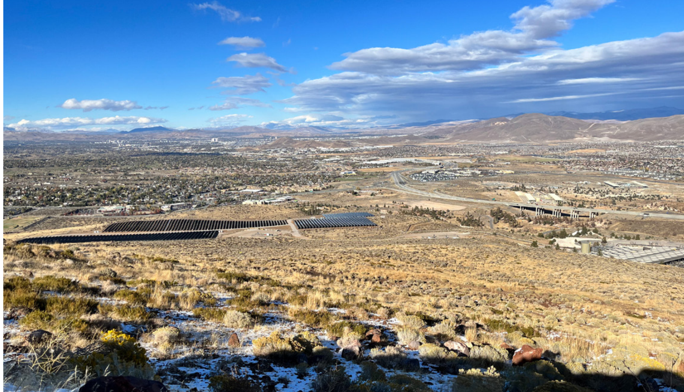
Geothermal Power Plant and Solar PV system, Steamboat Complex, NV, U.S.
