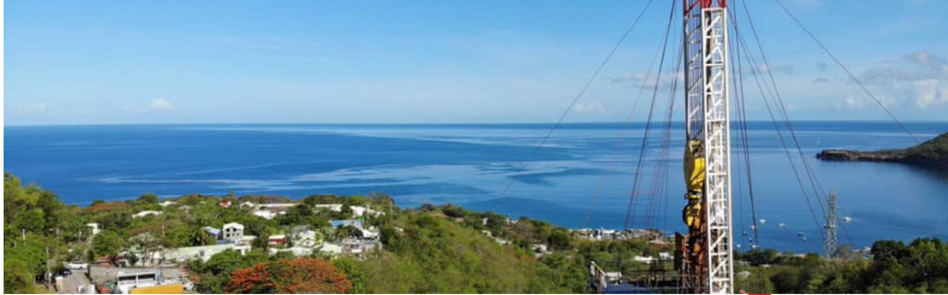
Drilling rig in Bouillante, Guadeloupe Island, France
