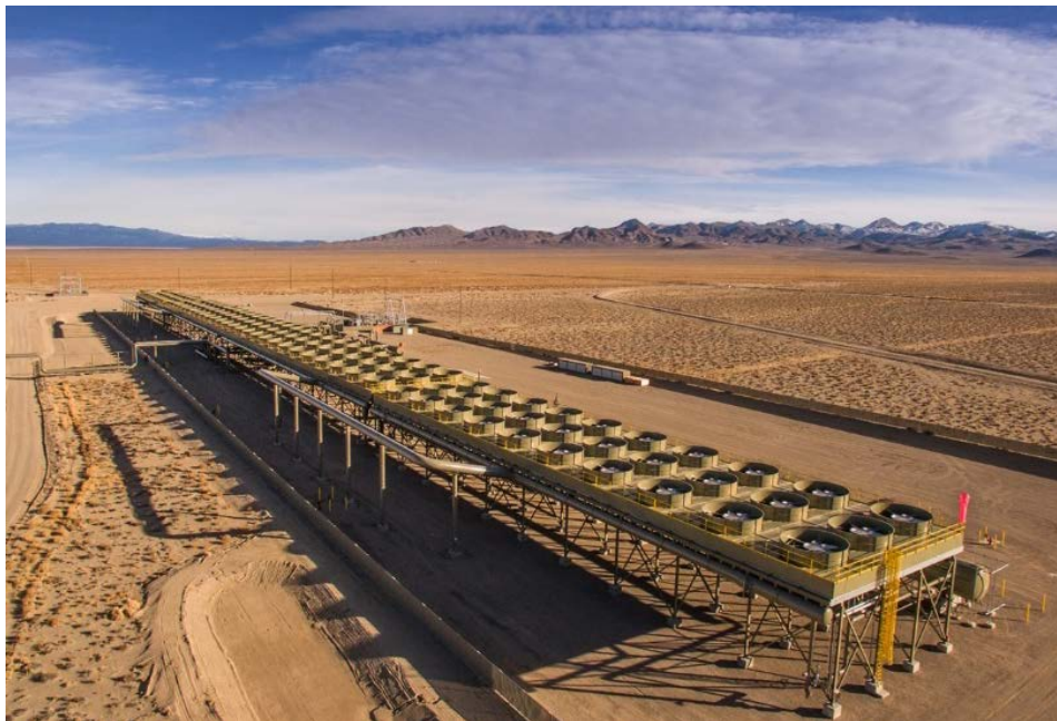
Figure 1 – Don A Campbell Air Cooled Condenser
