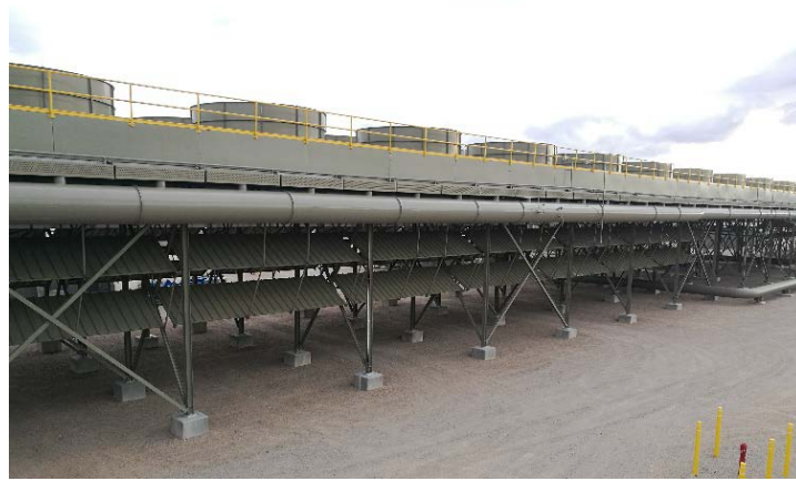
Figure 5 - WGV as install in DAC power plant ACC
